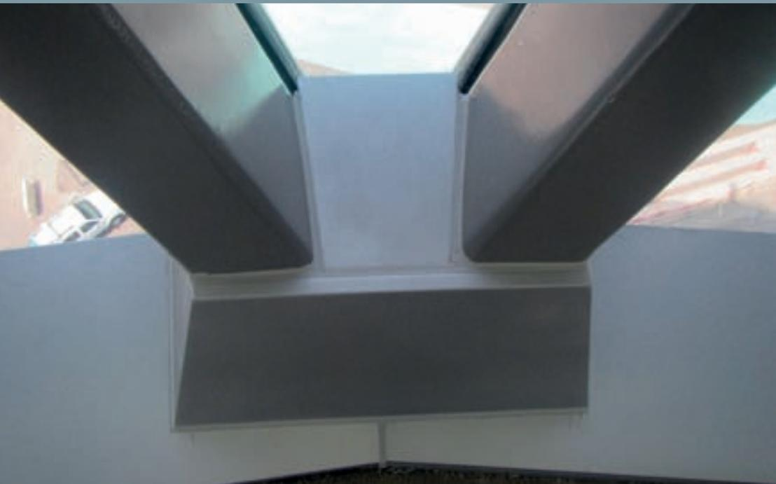
Yas Racetrack Shams Tower: Final application of corrosion protection of existing structure
